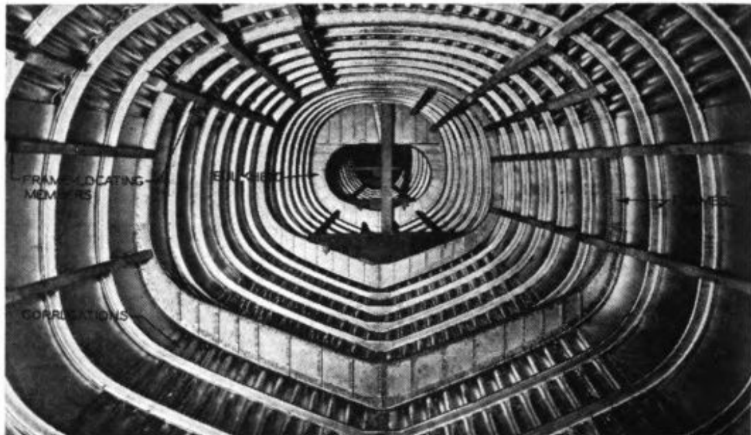
FIG. 36—INTERIOR OF FLYING-BOAT HULL
