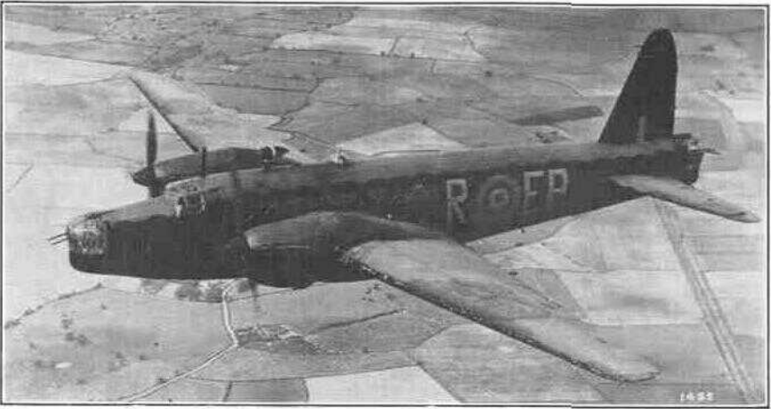
Photo. AI455. Vickers "Wellington" showing nose and tail-gun-turrets.
