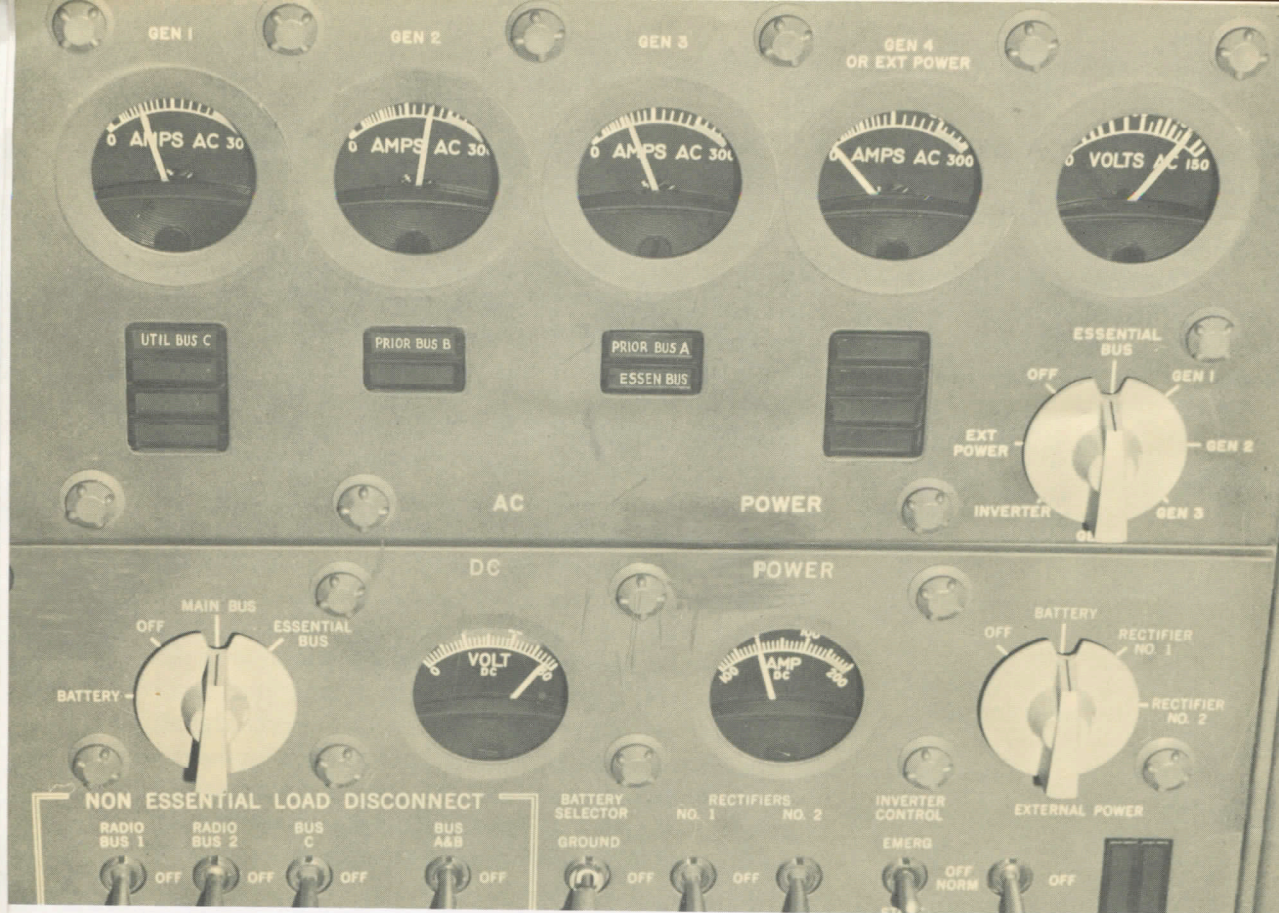
Figure 27 Overhead Electrical Control Panel
